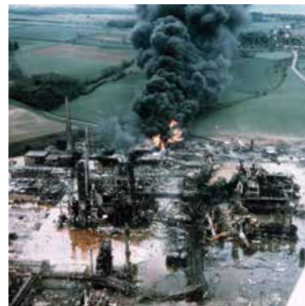
Fig 06: Vapour Cloud Explosion at Flixborough, U.K.
