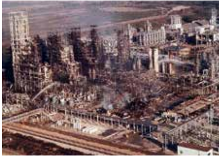
Fig 07: Vapour Cloud Explosion and Fireball at Philips Petroleum Chemical Complex, Pasadena.
