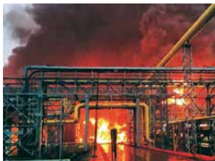
Fig 03: Fire at ONGC Gas Plant, Uran.
