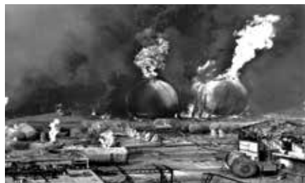
Fig 11: BLEVE at PEMEX LPG Bottling plant, Mexico City.
